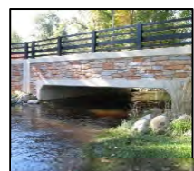
Figure 4: Three-sided box bridge
